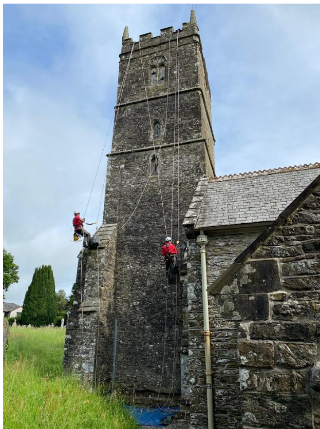
Wallwalkers rope access team re-pointing the tower
