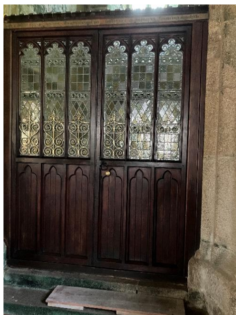
Restored Tower Screen doors
